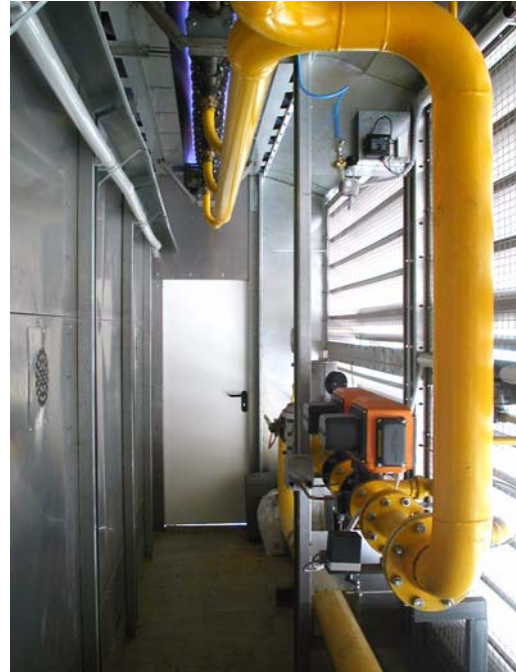
Direct air heating with NP-LE AIRFLO® burners in continuous flow dryers for grain
